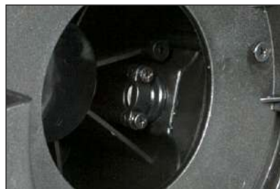
Internal cable fixing
